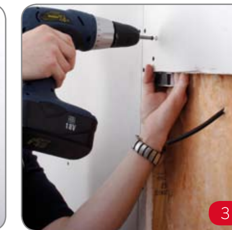
3 Fix installation lugs using two drywall screws secured through the front of the plasterboard into the plastic lug.
